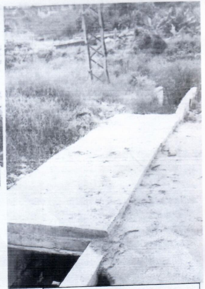
PIX. 1 - MECHANICS CULVET LEADING TO THE HIGH TENSION
